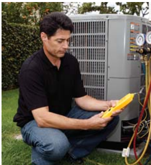
The Air Conditioning Refrigerant Charge Test checks your unit's performance so that you can maximize indoor comfort levels.
